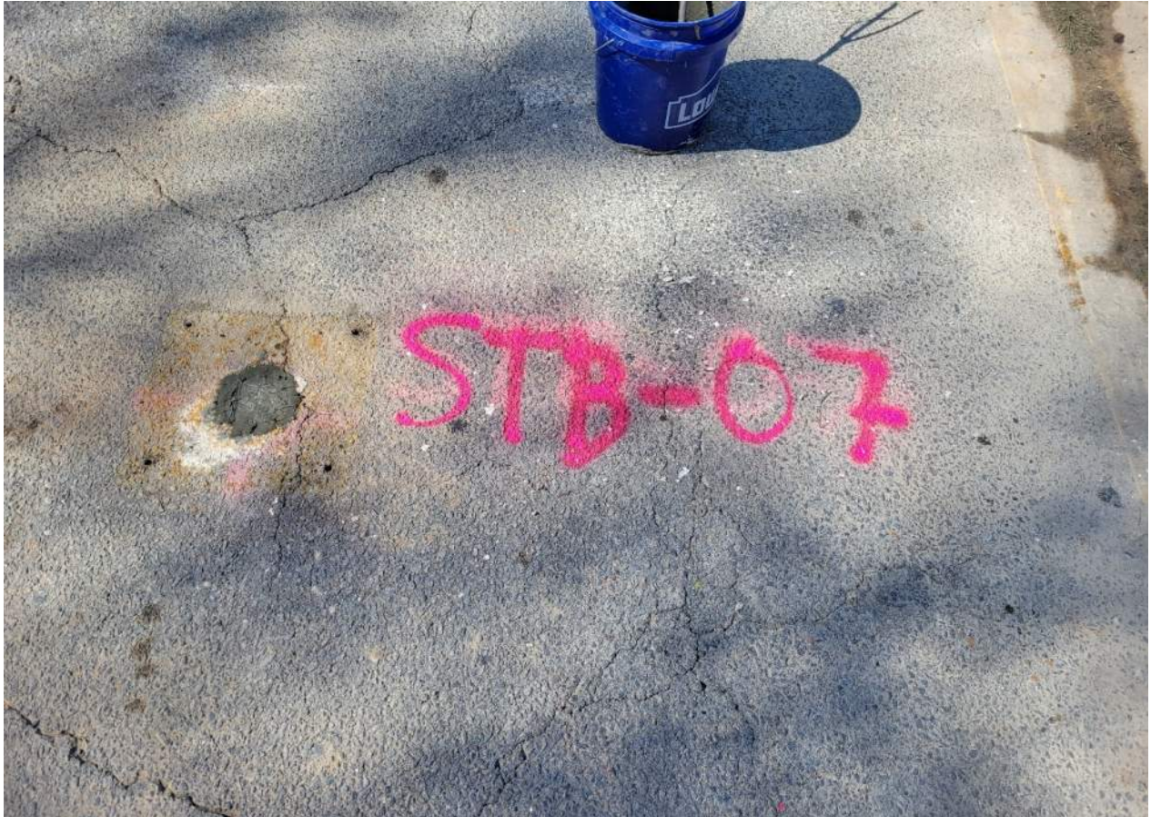
Photograph 7: STB-07 (After Drilling)
