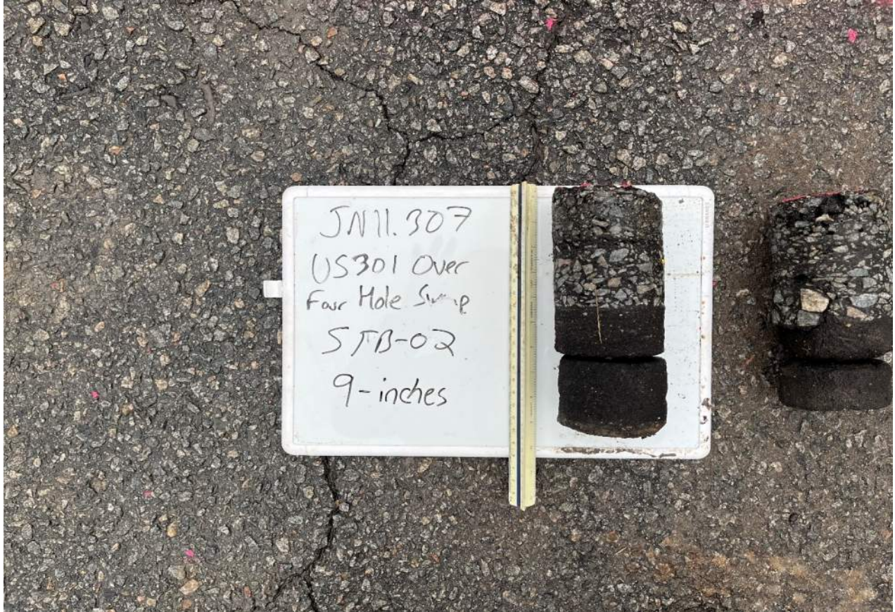
Photograph 2: Asphalt Core STB-02
