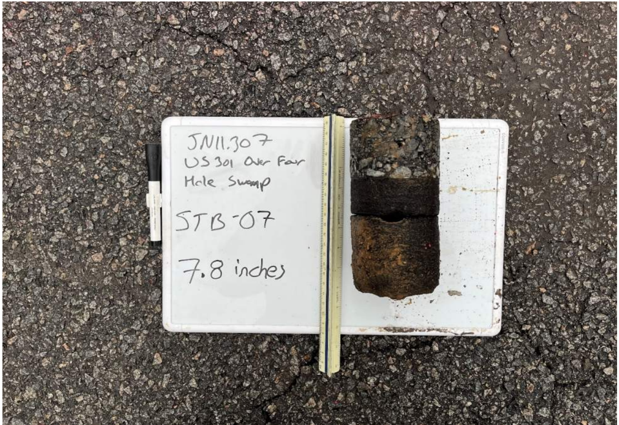
Photograph 4: Asphalt Core STB-07
