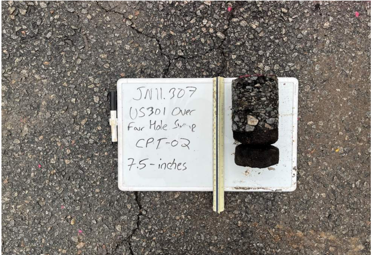
Photograph 6: Asphalt Core CPT-02
