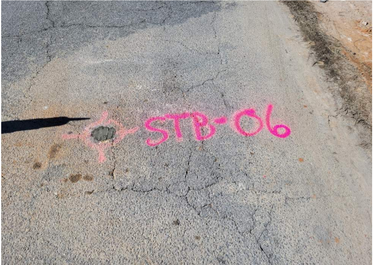
Photograph 6: STB-06 (After Drilling)
